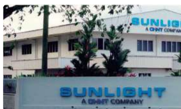
Sunlight Singapore & Malaysia Main Products: Low-voltage Switchgears
