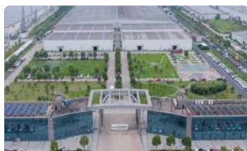
Haining Solar Intelligent Factory
