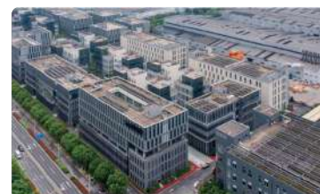
Power T&D Shanghai Factory
