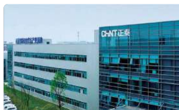
Power T&D Jiaxing Factory
